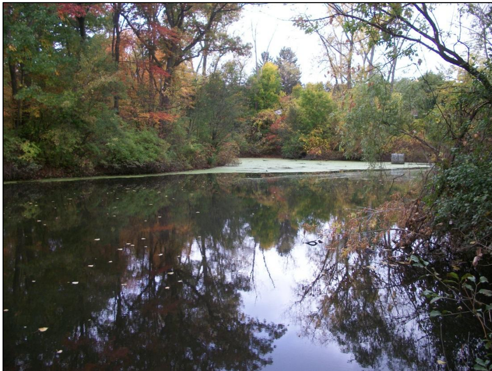
Site Photo 12: Stilling basin (drainage structure visible)
