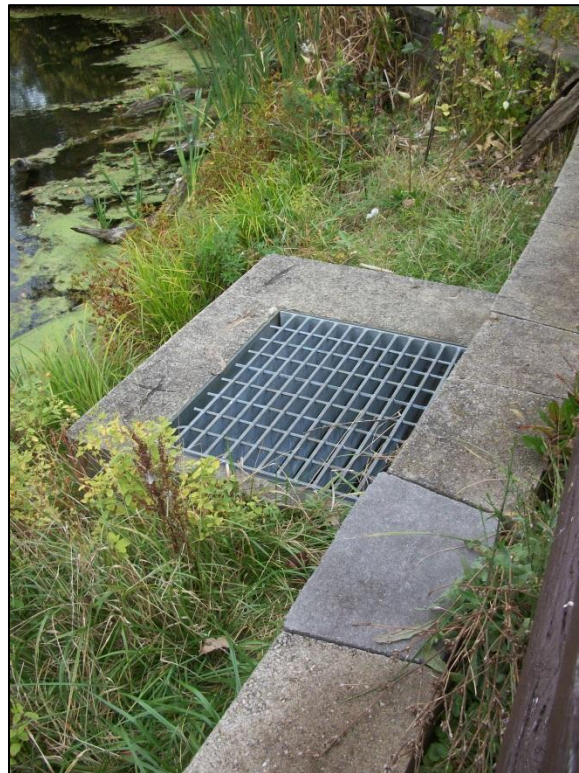
Site Photo 16: Pond overflow structure
