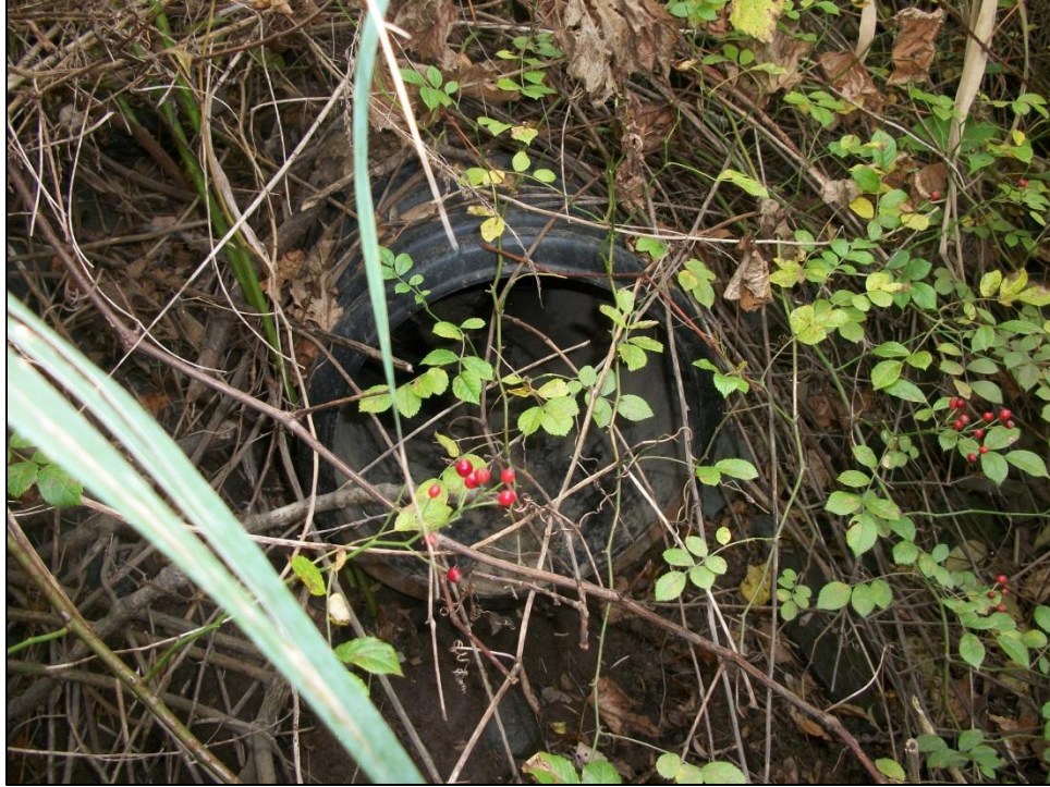
Site Photo 5: Culvert in southwest corner of stilling basin
