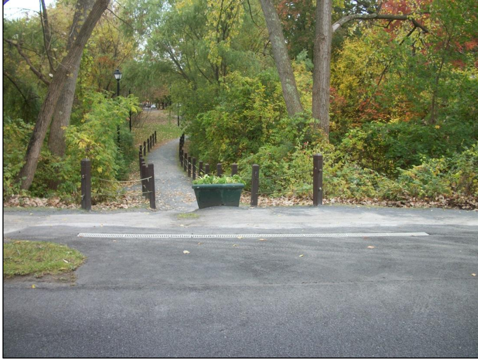
Site Photo 9: Trench drain on northeast end of pond (near walking trail)
