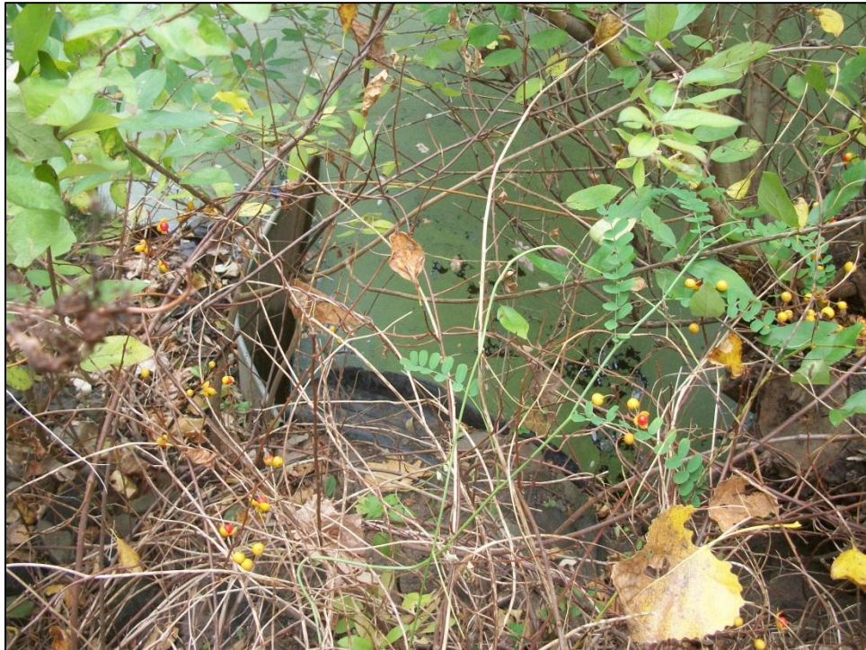
Site Photo 6: Culvert in southeast corner of stilling basin
