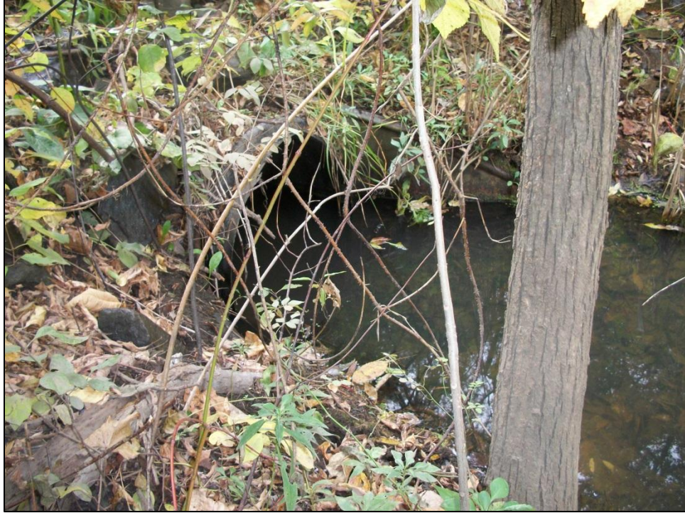
Site Photo 3: Culvert in southwest corner of stilling basin
