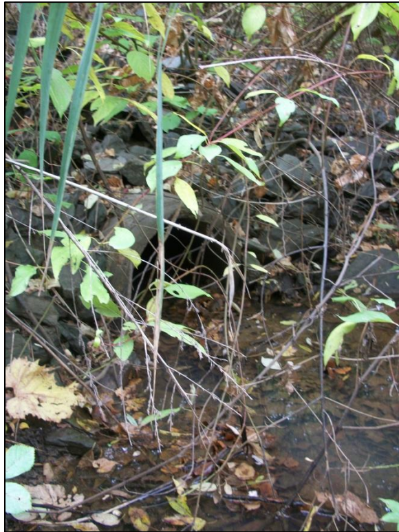
Site Photo 4: Culvert in southwest corner of stilling basin
