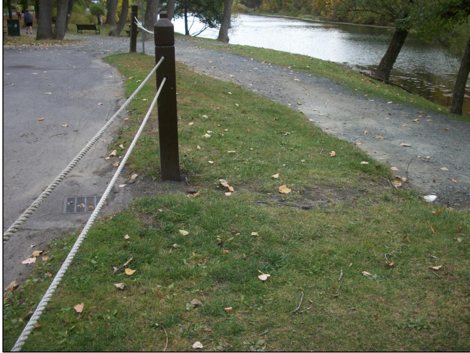
Site Photo 7: Catch basin and outlet from parking lot
