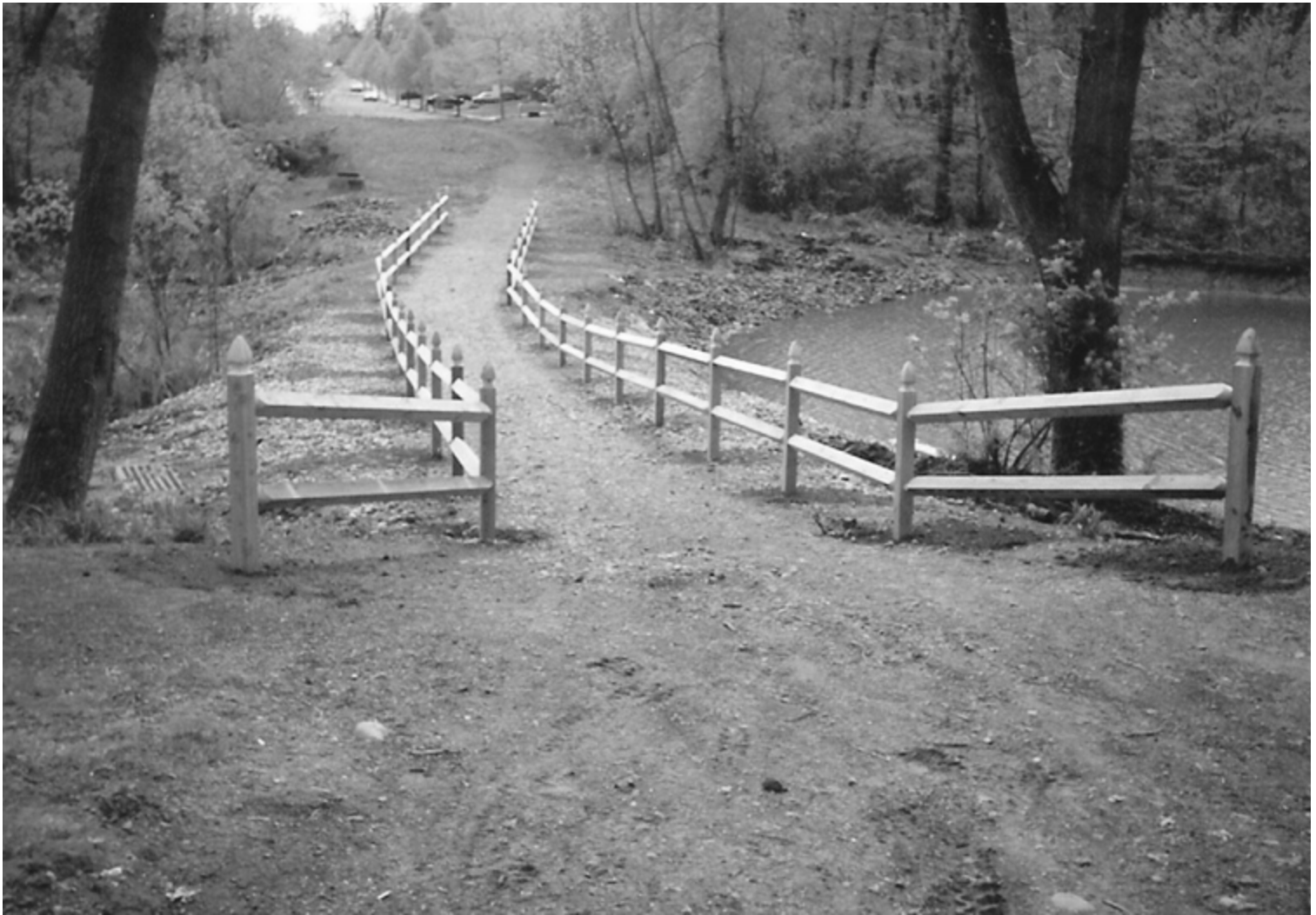
New fence and trail complete
