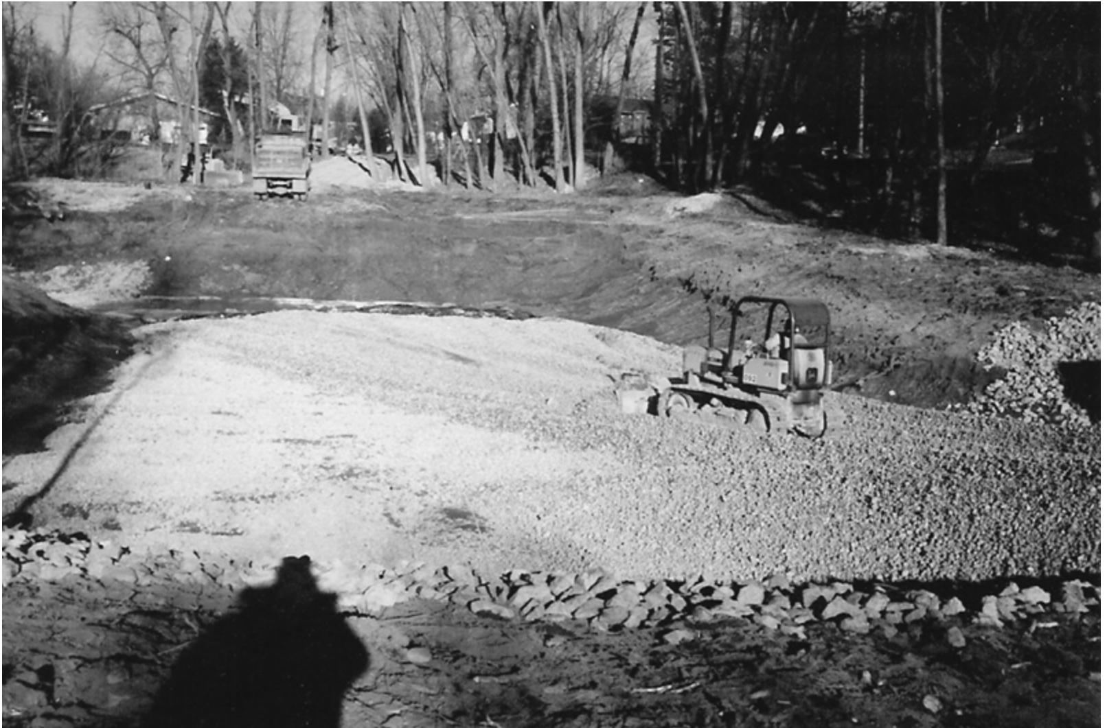
Placing of fine stone layer over rip-rap in stilling basin
