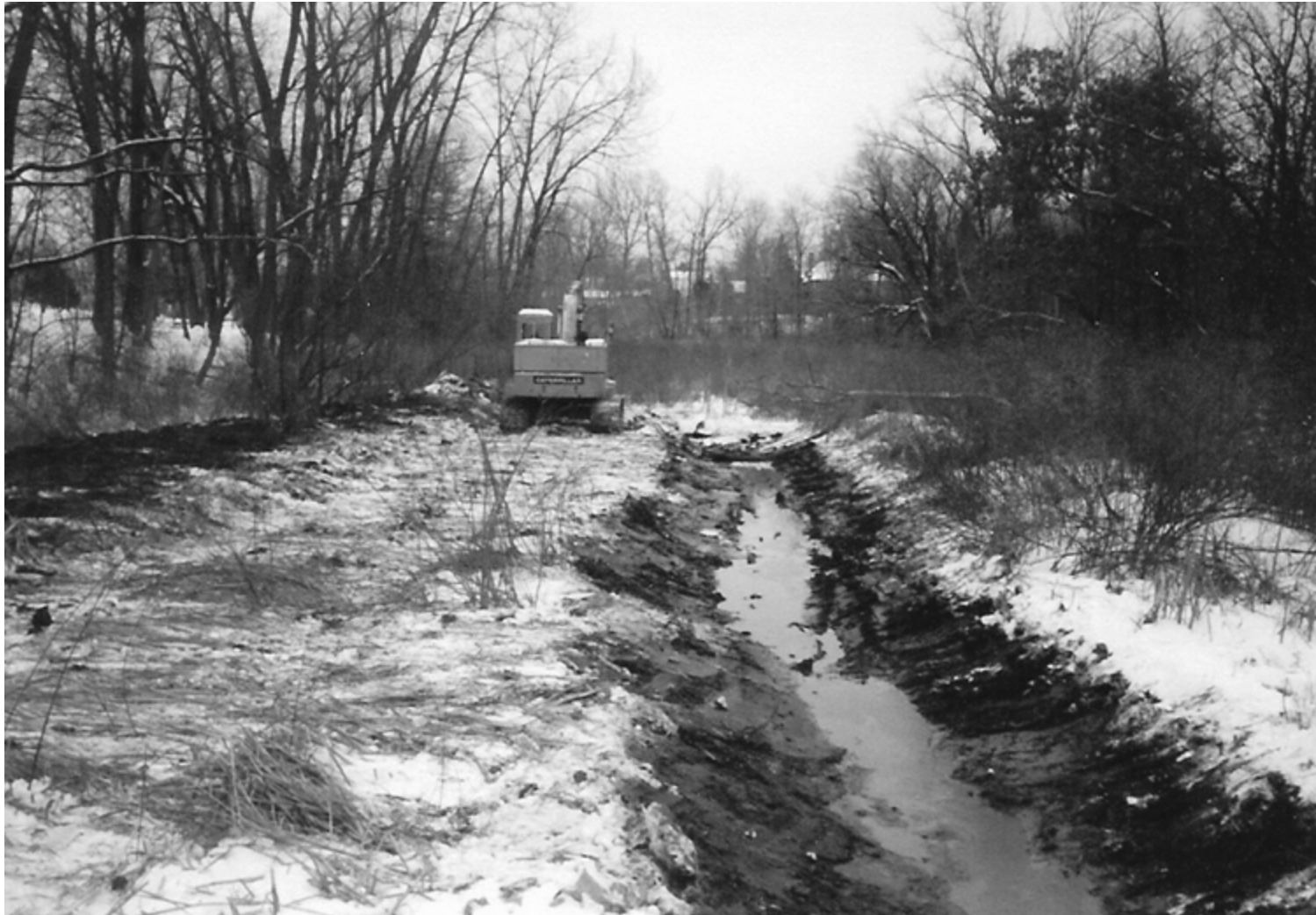
Excavation of trench connecting stilling basin to main pond
