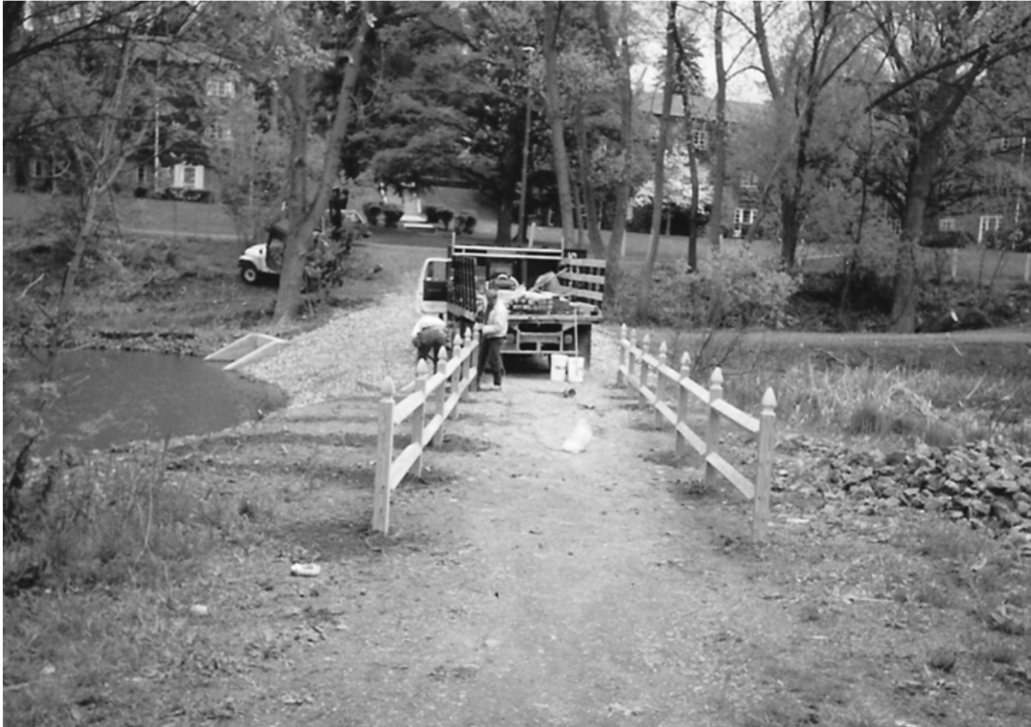
Installing new fence and trail
