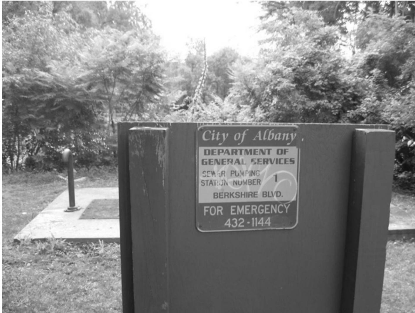
View of Pump Station from Davis Avenue. 7/1/2009
