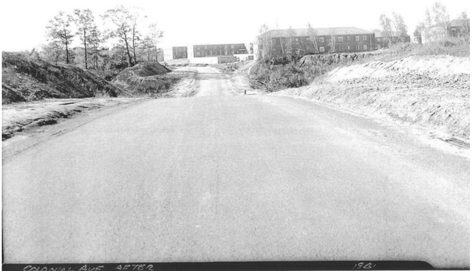
Photo showing Colonial Avenue after construction in 1941
