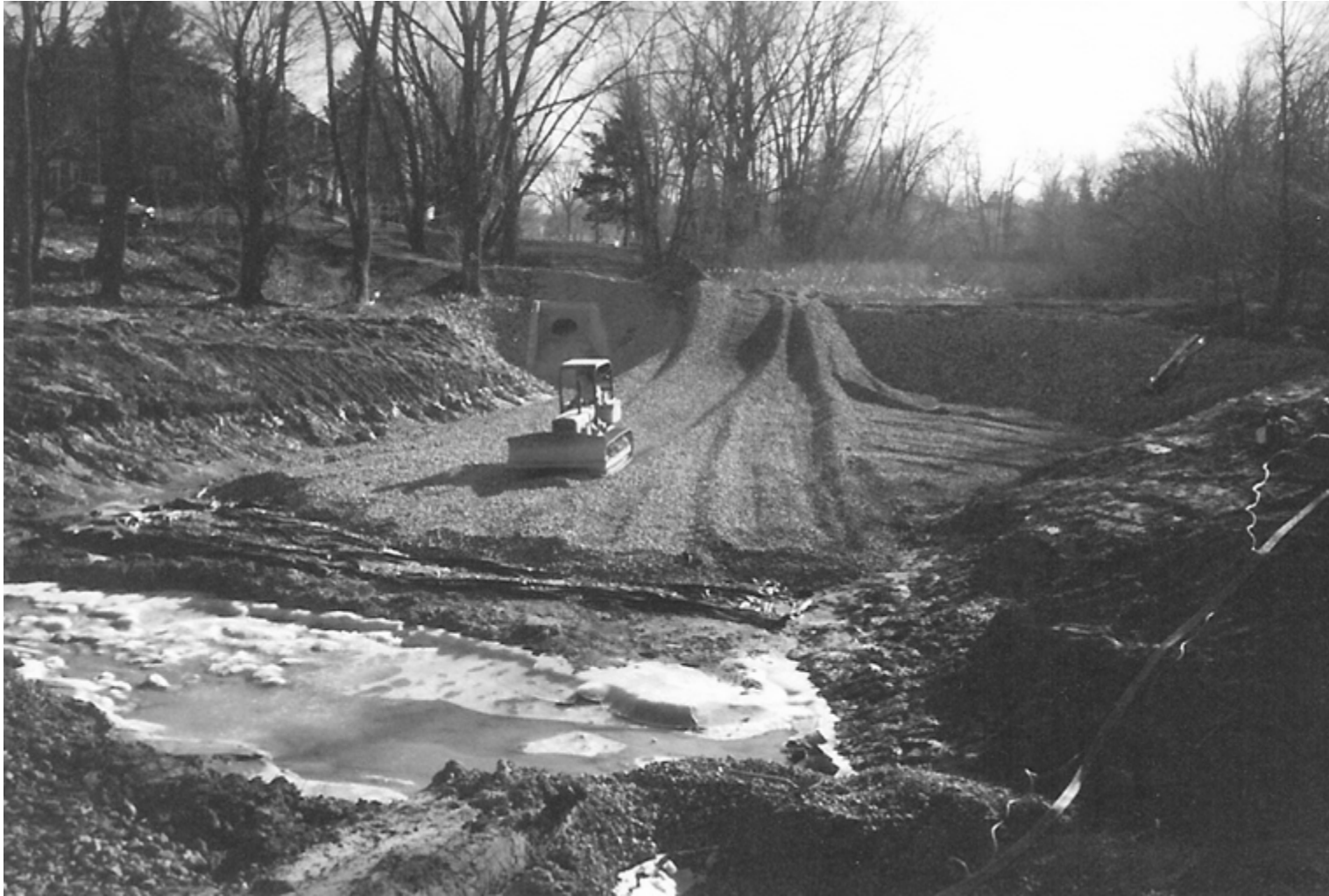
Placing of rip-rap layer in stilling basin
