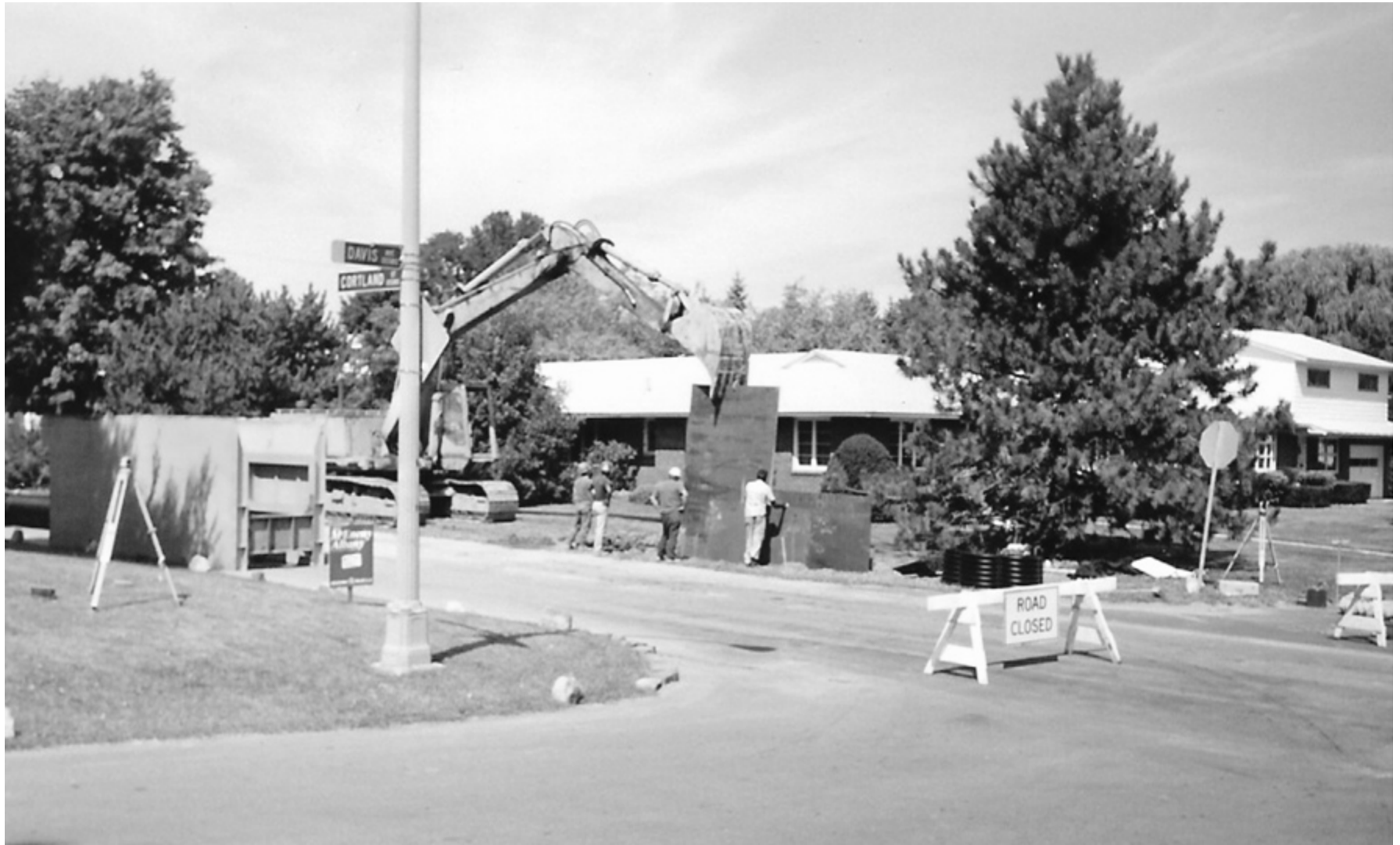
Installing new storm sewer by Davis Avenue & Cortland Street
