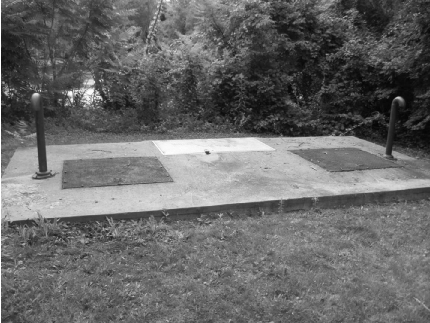
View of Top of Pump Station . 7/1/2009
